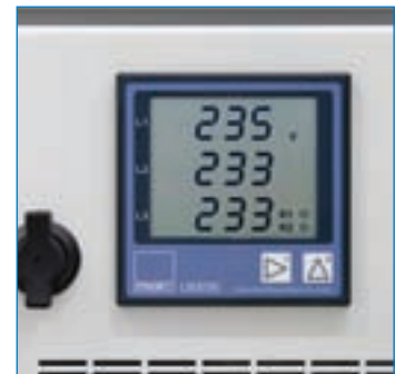
Outgoing unit with digital measurement
