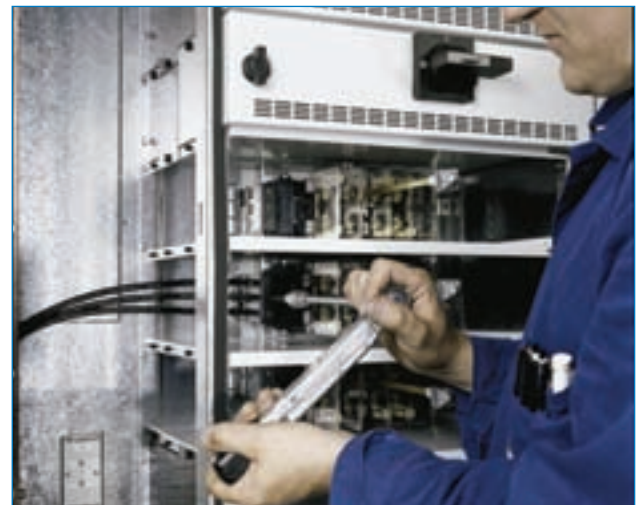
Rotary handle operated MCCBs and fused switches
